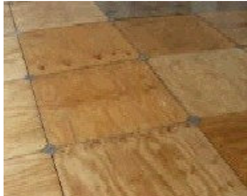
Laydown Plywood Flooring
